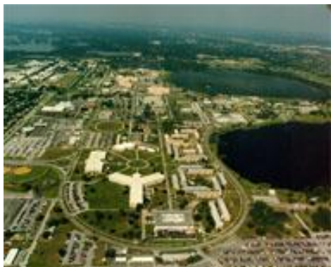
Aerial of NTC Main Base
