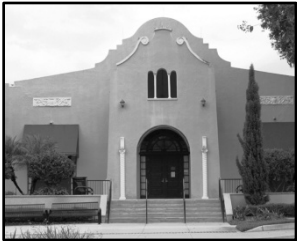
Marks Street School
