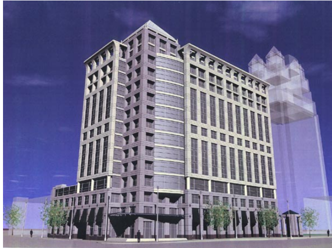
The Lincoln Office Building at the northwest corner of Orange Avenue and South Street is just one of many buildings under construction.
