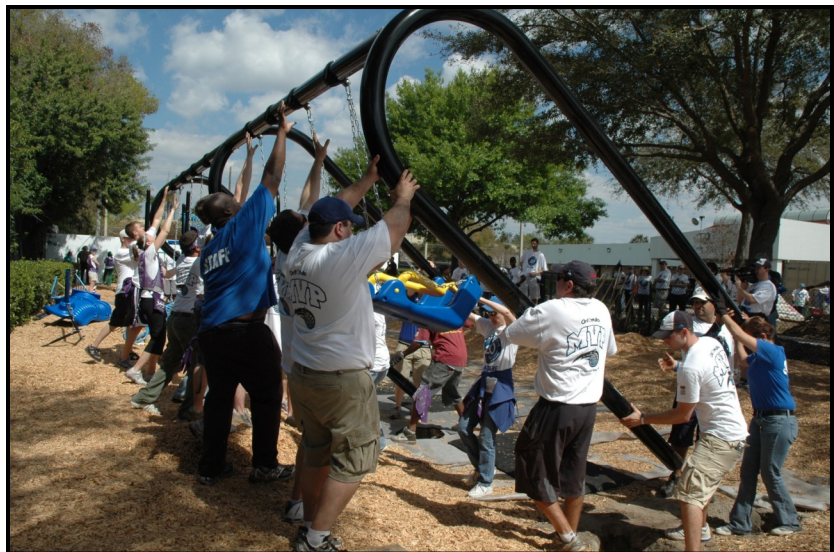
Building a KaBOOM! playground at the Jackson Center.
