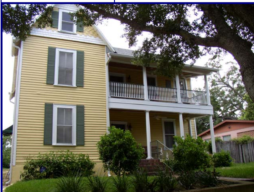
Front Elevation of Subject Property.
