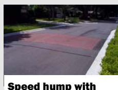
Speed hump with brick-colored textured asphalt
